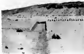
Figure 77. Here is a view of decoy dragon's teeth and a decoy antimechanized ditch. A camouflaged real ditch is on the foreground, covered with wire netting, cloth, and sand.
